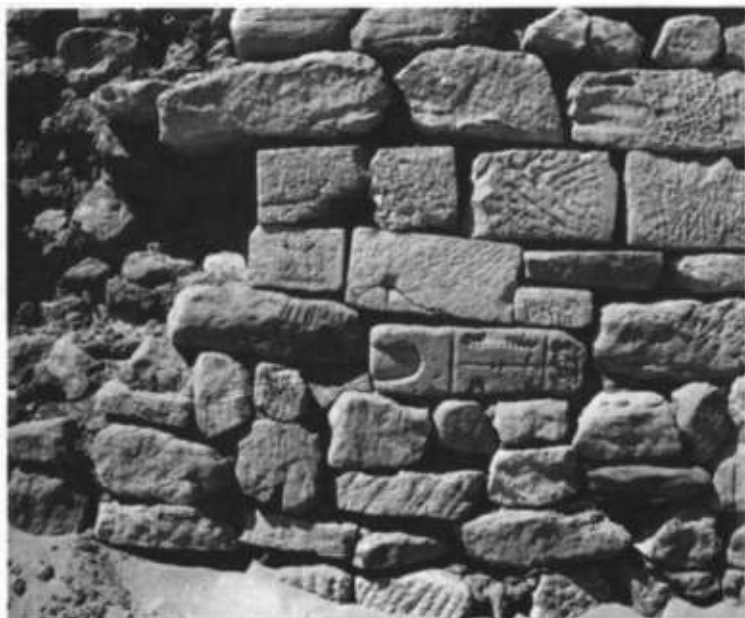
PLATE 16.2 The city wall of the Arab citadel of Faras, reconstructed with ancient bricks
