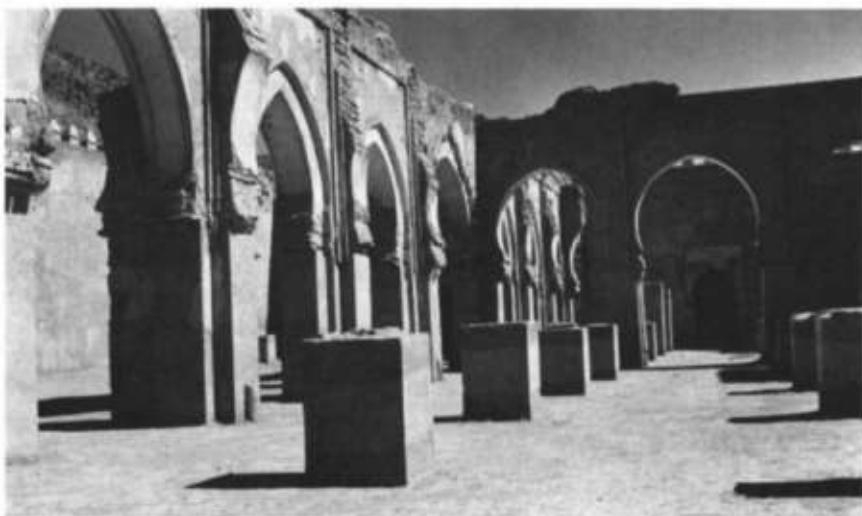
PLATE 2.2 The inner courtyard of the mosque at Tinmallal
