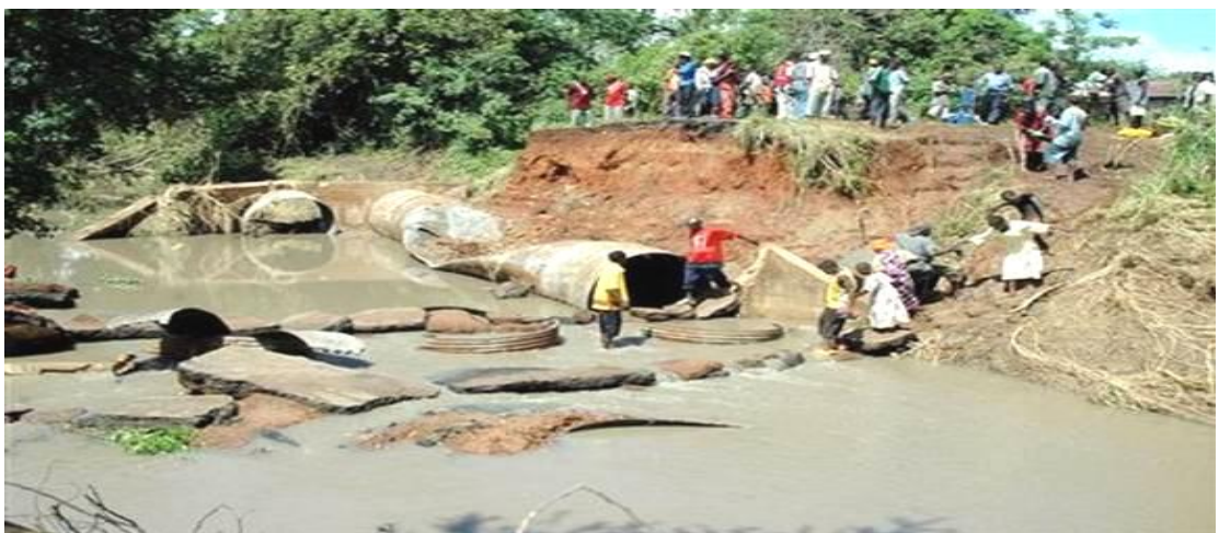
Figure 4.16: Effect of Floods on Infrastructure (Bridge at Msambweni Village - Tanga to Mombasa Road)
