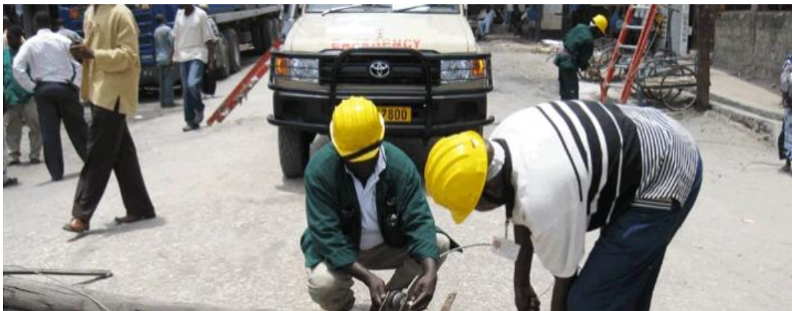
Photo 6.1: TANESCO Emergency Team at site (2009)
