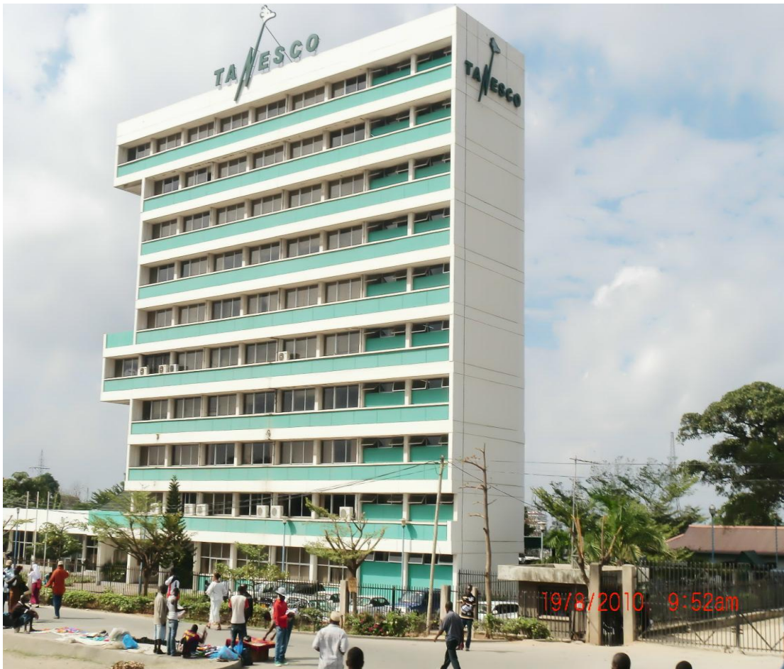
Photo 1: TANESCO Headquarters in Dar es Salaam, Tanzania
