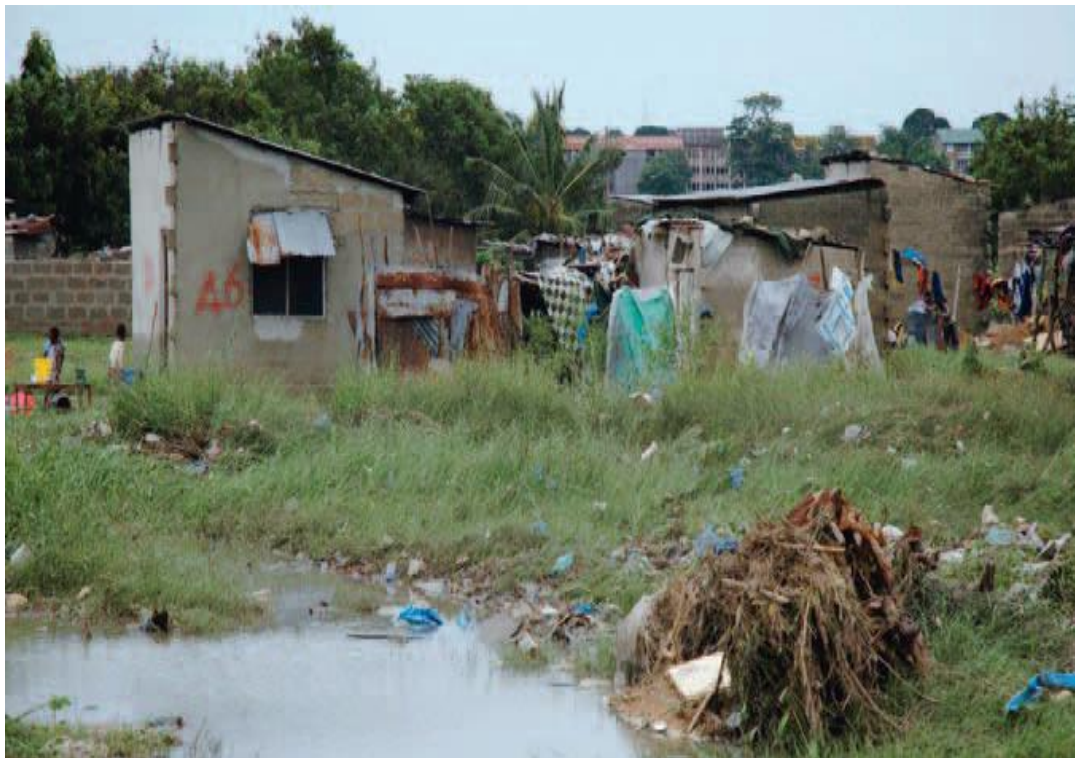
Figure 4.1: Photograph Showing Settlement blocking drainage system
