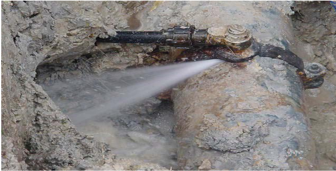
Figure 1.1: Water Leakage Due to Aged Water Supply System
