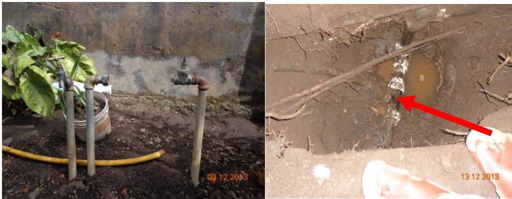
Figure 4.8 Unauthorized Water Connection in some Customers' Premises
