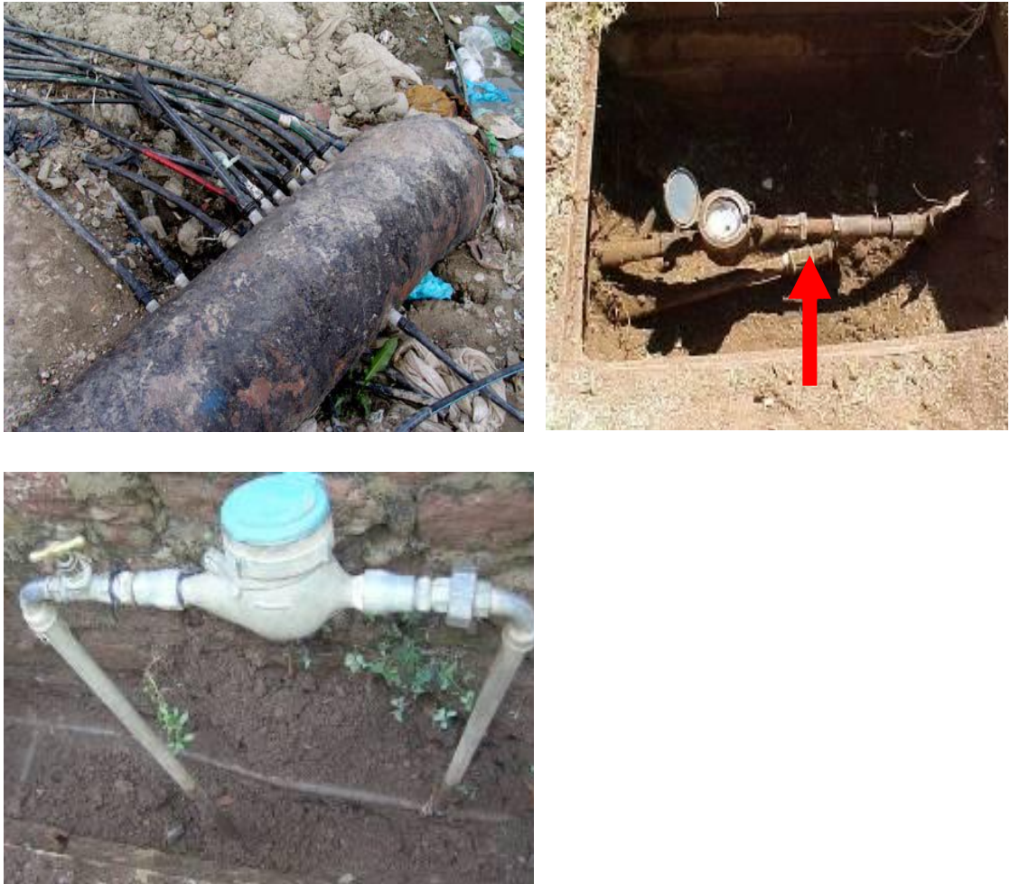
Figure 4.10 Illegal Connections
