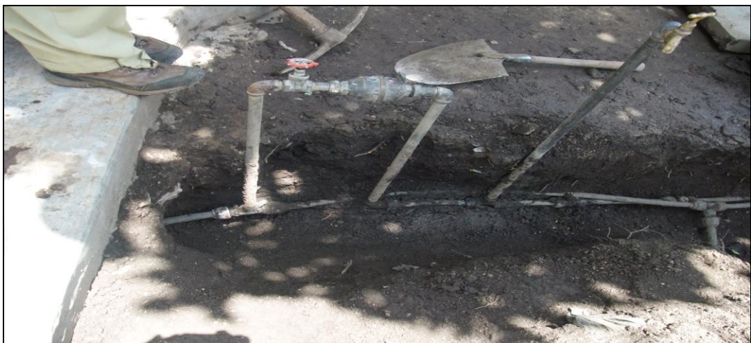
Figure 2.3: Meter by-pass
