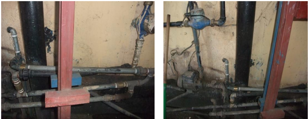
Poor connections
