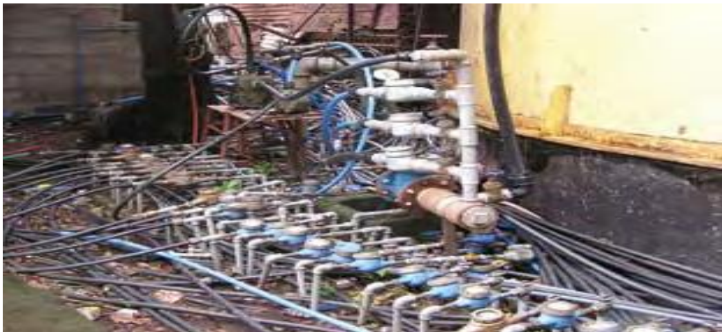
Figure 2.2 Multiple Connections
