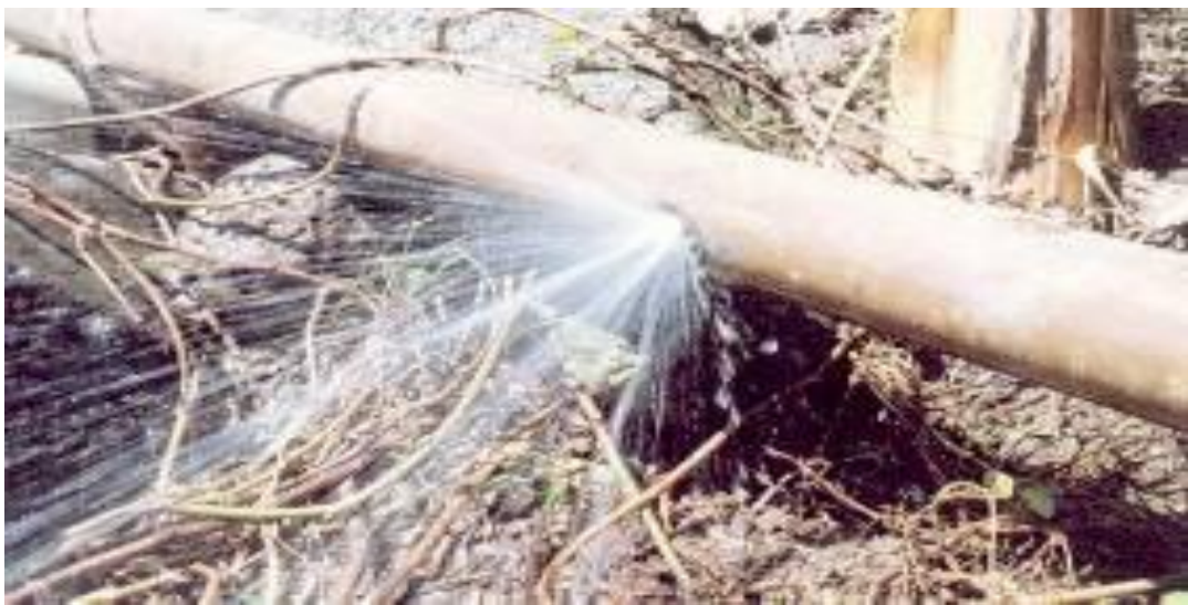
Figure 4.6: Water Leakage Due to High Pressure
