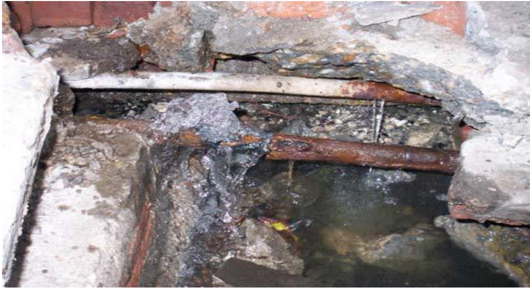
Figure 4.5: Old Piped System Increase Leakage of Water Supply
