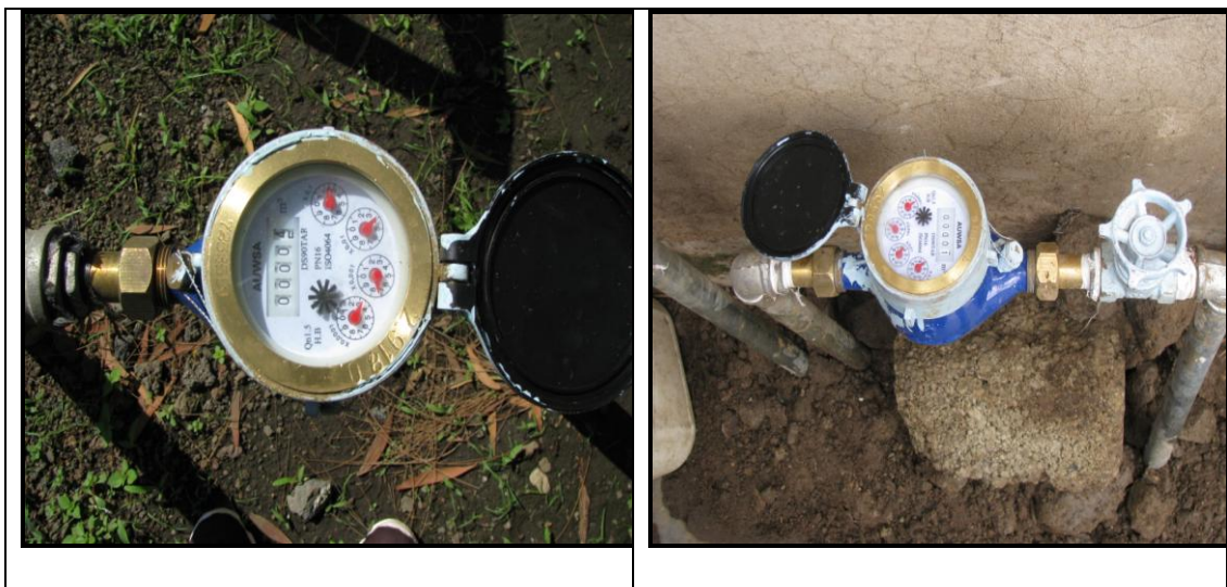
Figure 4.12: Meter System for Customers and Water Sources
