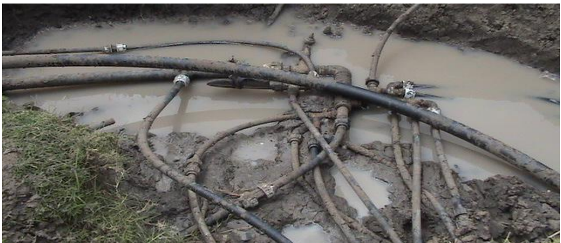
Figure 2.1 Multiple Illegal Connections with Massive Leakage
