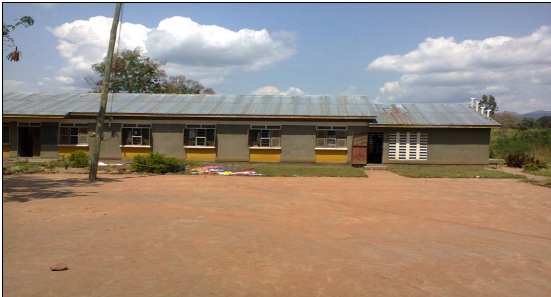
Plate 4.3: Mikumi Secondary School, Female Hostel which was built by MINAPA
