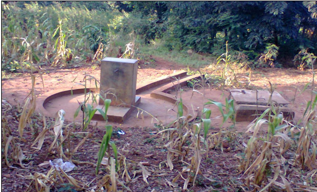
Plate 4.2: The Water Supply Project at Mikumi Mpya Primary School Which Was Built by MINAPA
