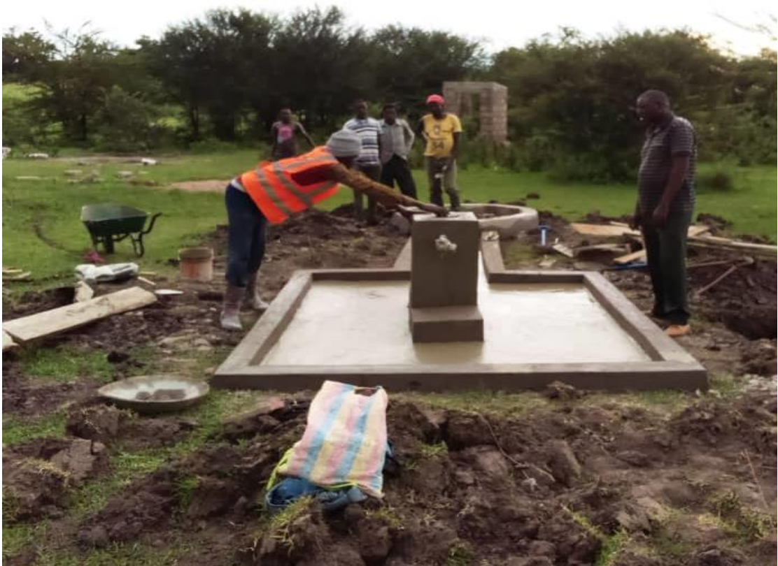
Plate 4.3: Rehabilitation of Shallow Wells at Bulamba Village
