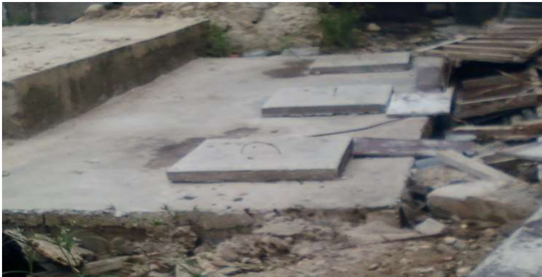
Plate 4.3: Wastewater separation tank
