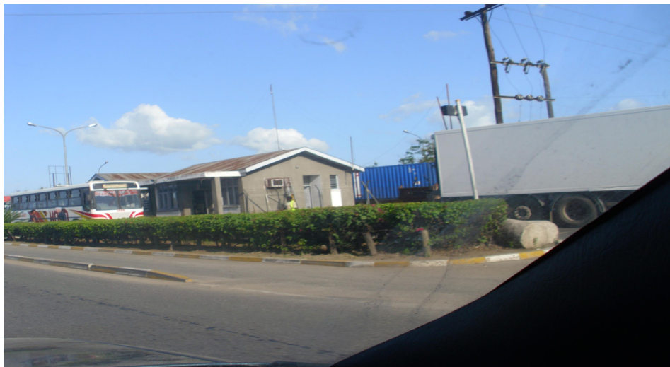
Figure 1: Kibaha Weigh Bridge
