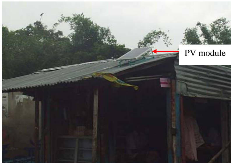
Figure 9: Roof-house PV module mounting.
