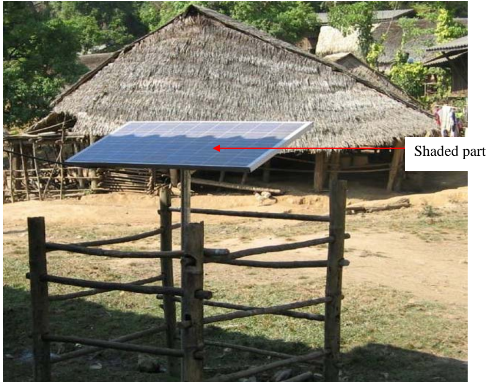
Figure 10: Wrong installation place of the PV module
