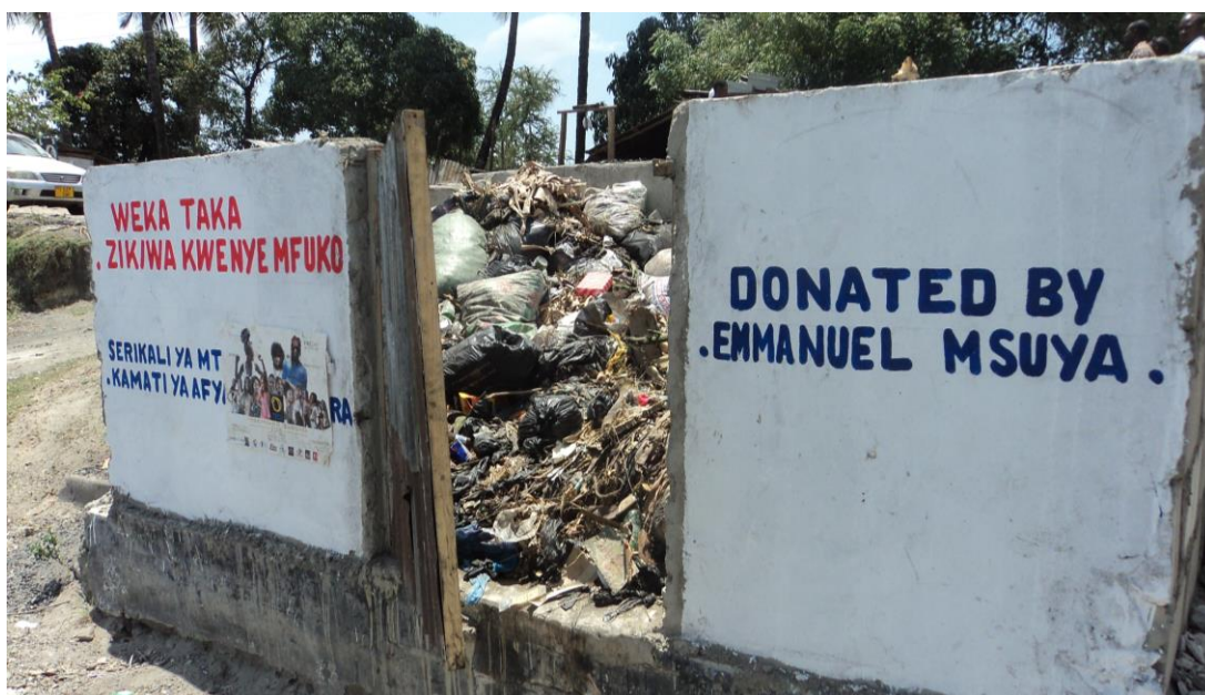
Figure 4.5: Newly Built Dumping Collection Point
