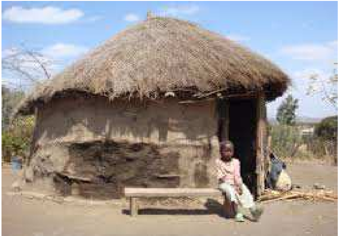
Figure 4.7: A Boma Built on Locally Procured Materials Including Mud, Wood and Roofed on Thatch at Uwiro
