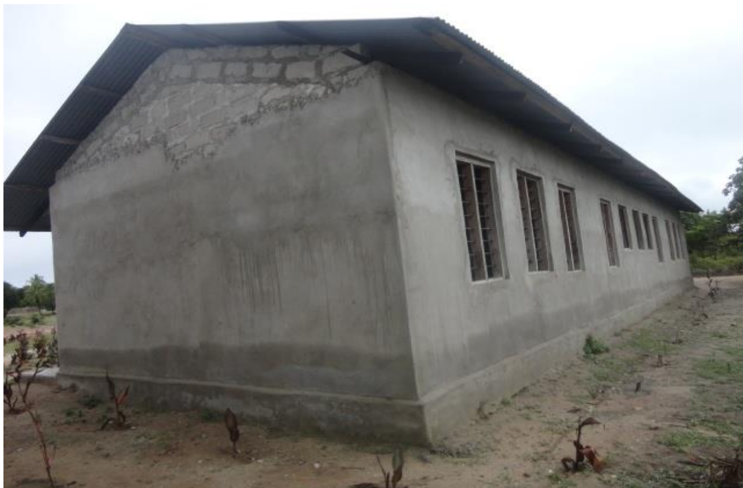
Figure 4.1: Classrooms being Constructed by SEDP at MACEHU Secondary School
