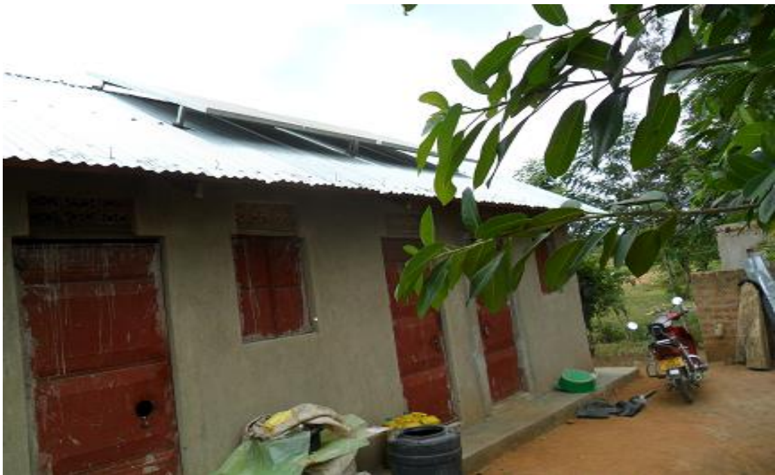
Figure 3.2: System installed in Budaka, Eastern Uganda in November 2012
